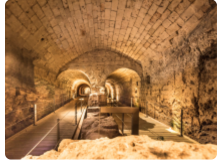
The 350 meters long Templars tunnel leads from the Templars Palace up to Akko port in the east, Akko, Israel
